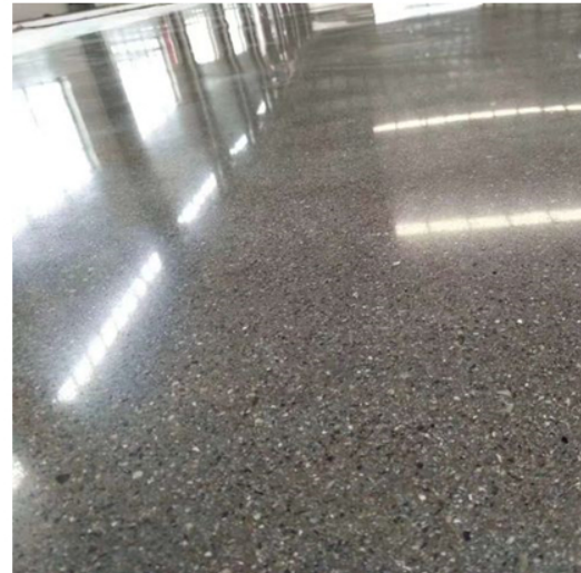
After Grinding and Polishing
