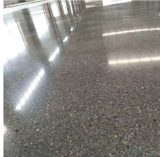
After Grinding and Polishing
