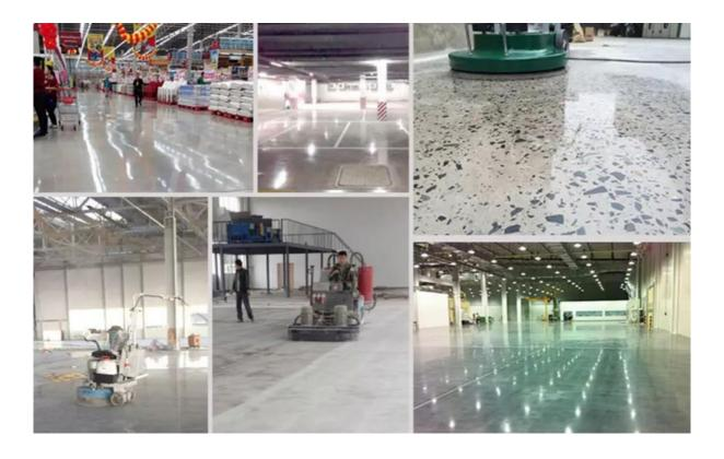
Metal bond diamonds high grinding efficiency and low grinding force generates less heat in the grinding process.
