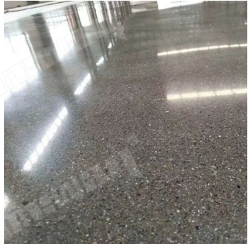
After Grinding and Polishing
