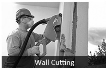
Concrete With Rebar Cutting
