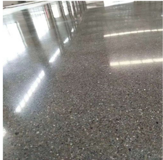
After Grinding and Polishing
