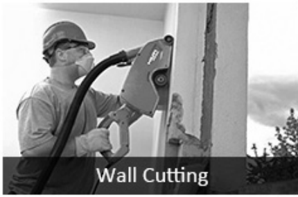
Concrete With Rebar Cutting
