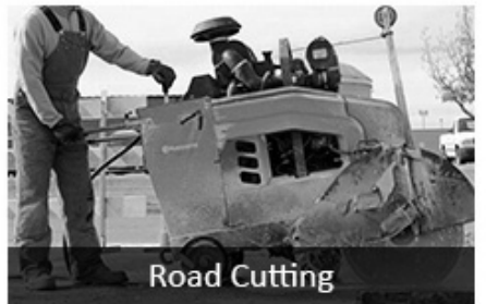
Concrete With Rebar Cutting
