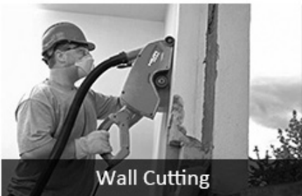
Concrete With Rebar Cutting
