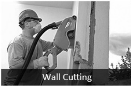
Concrete With Rebar Cutting
