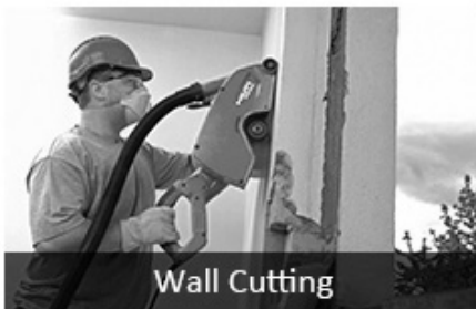
Concrete With Rebar Cutting
