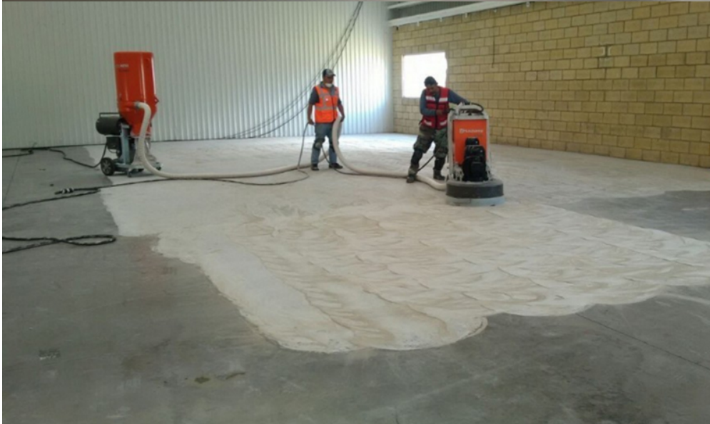
Concrete Grinding Effect
