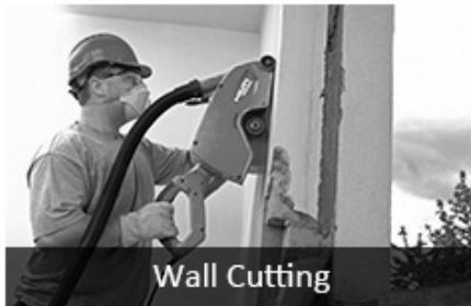
Concrete With Rebar Cutting
