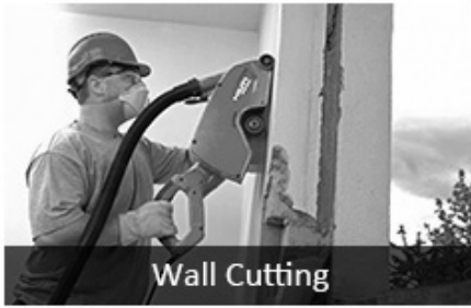
Concrete With Rebar Cutting
