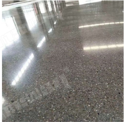
After Grinding and Polishing
