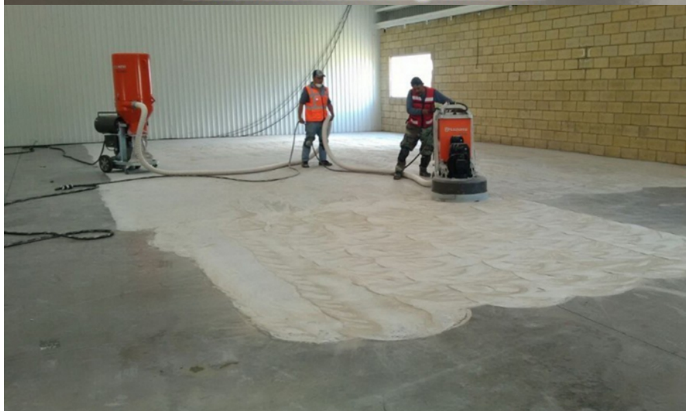
Concrete Grinding Effect
