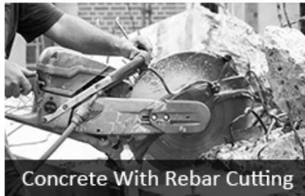
Concrete With Rebar Cutting
