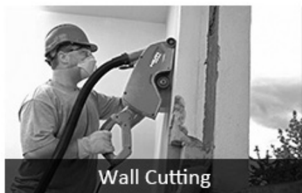
Concrete With Rebar Cutting
