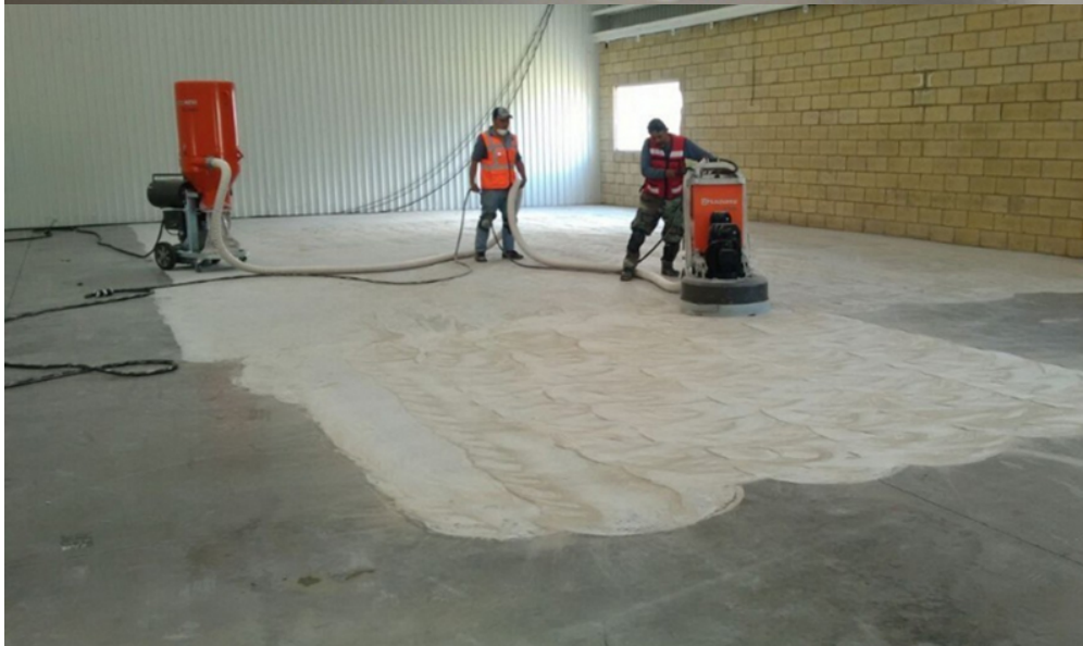
Concrete Grinding Effect
