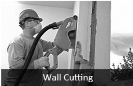
Concrete With Rebar Cutting
