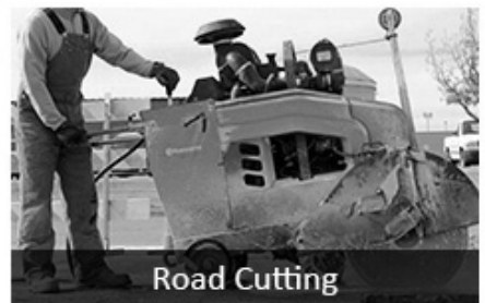
Concrete With Rebar Cutting
