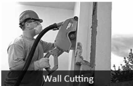
Concrete With Rebar Cutting
