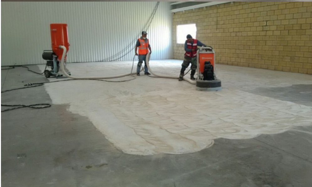
Concrete Grinding Effect
