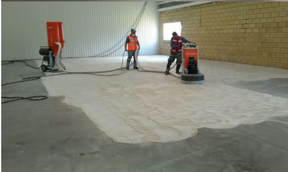
Concrete Grinding Effect
