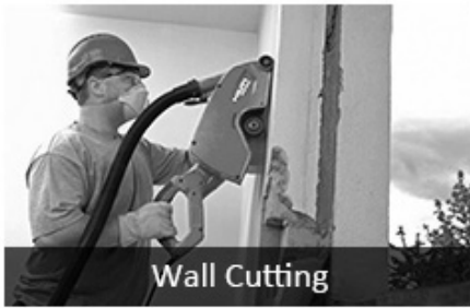
Concrete With Rebar Cutting
