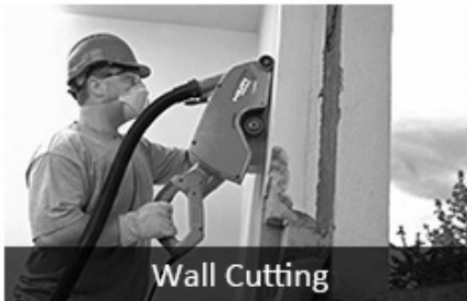
Concrete With Rebar Cutting
