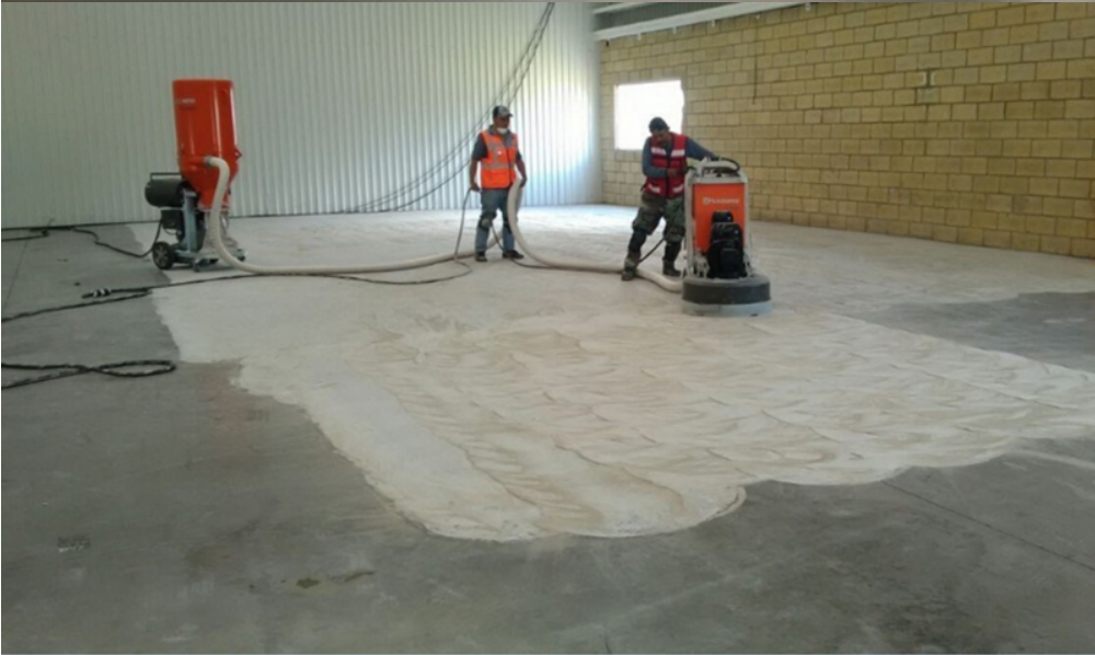
Concrete Grinding Effect
