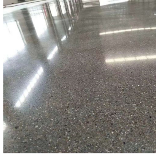
After Grinding and Polishing
