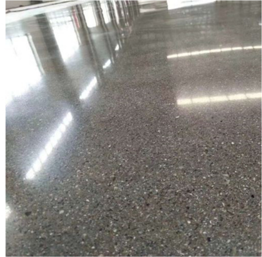
After Grinding and Polishing
