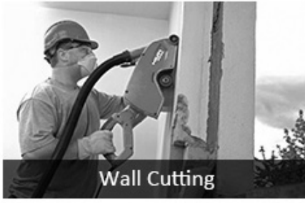
Concrete With Rebar Cutting
